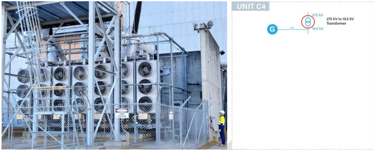
Figure 45 Unit C3 generator transformer (identical to Unit C4)
