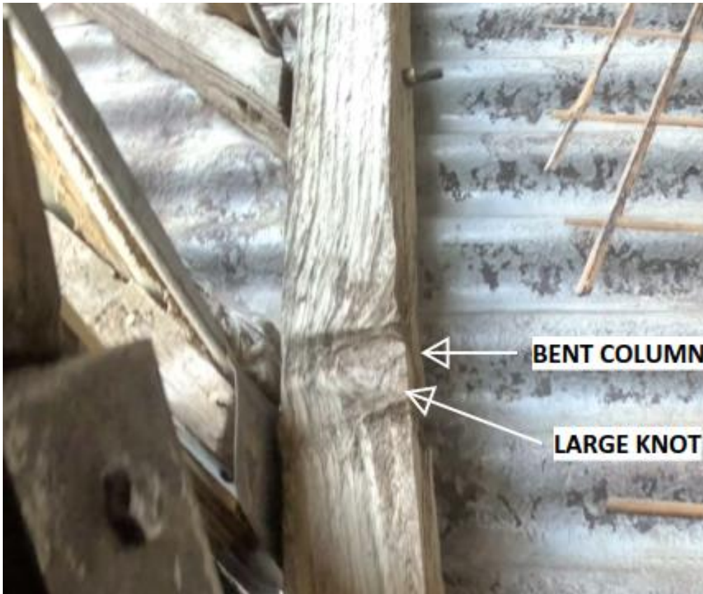
Figure 7.17 Bent end wall column - unknown location
