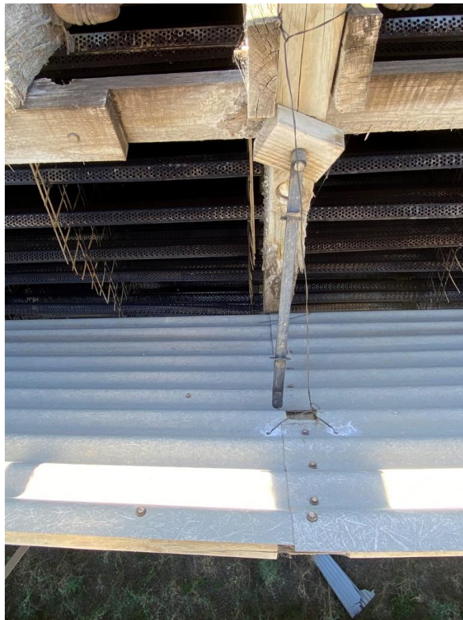
Figure 5.18 Typical temporary repair to re-support louvre supports using wire ties
