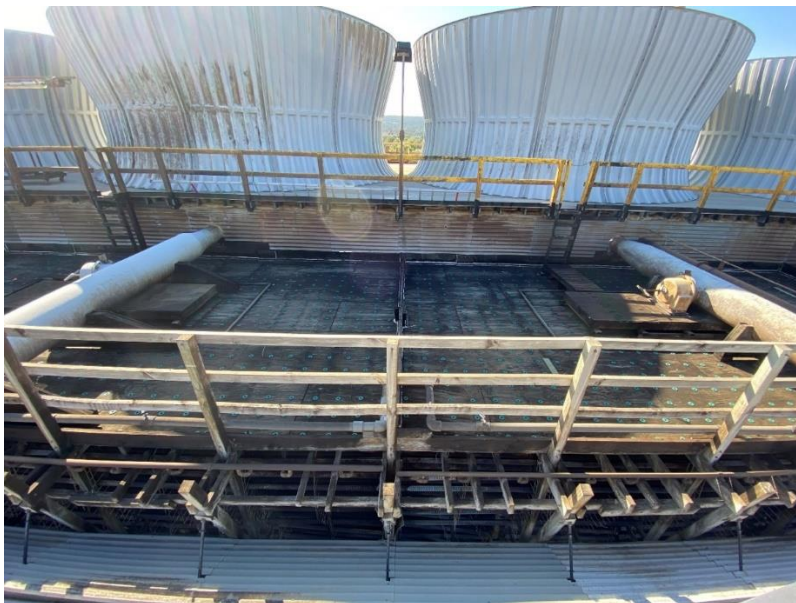
Figure 5.25 Hot water basin appeared to be in reasonable condition
