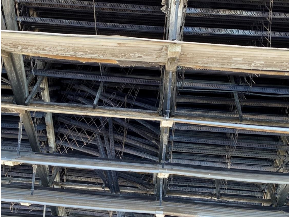
Figure 5.22 Some sections of fill collapsed though not widespread on this side of CT4
