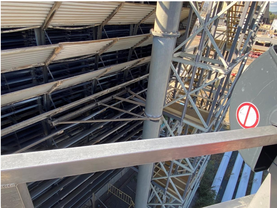
Figure 5.14 Steel brace configuration for riser pipes
