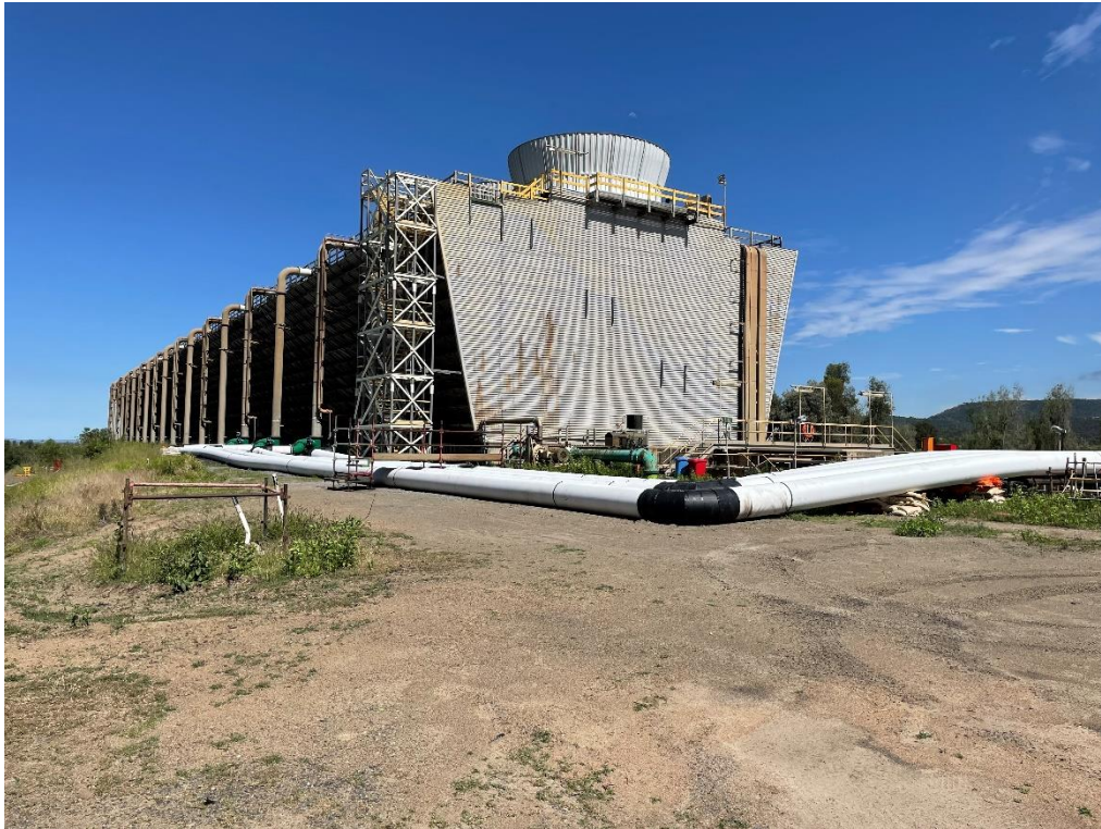
Figure 1.3 Cooling Tower CT4 viewed from the south-east
