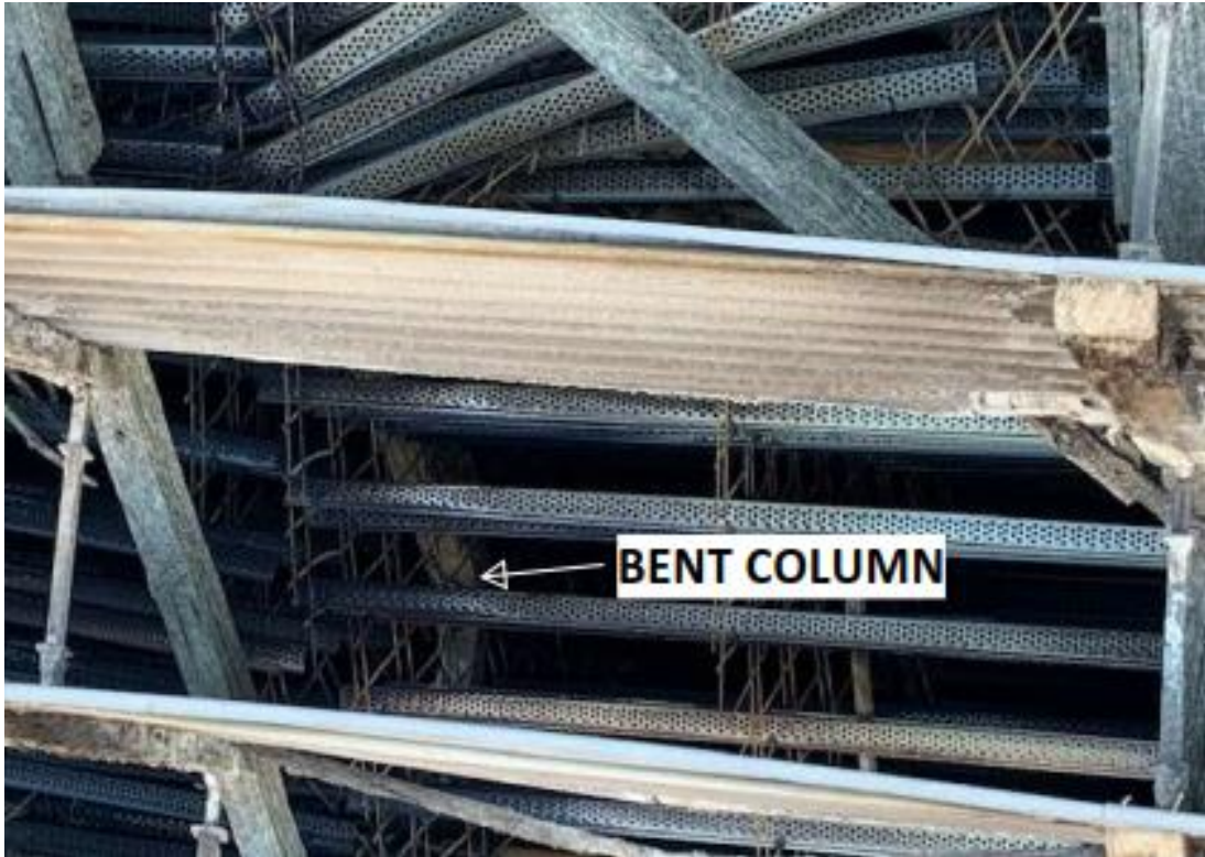
Figure 7.11 Bent Column CT3 unknown location - Marley April 2022
