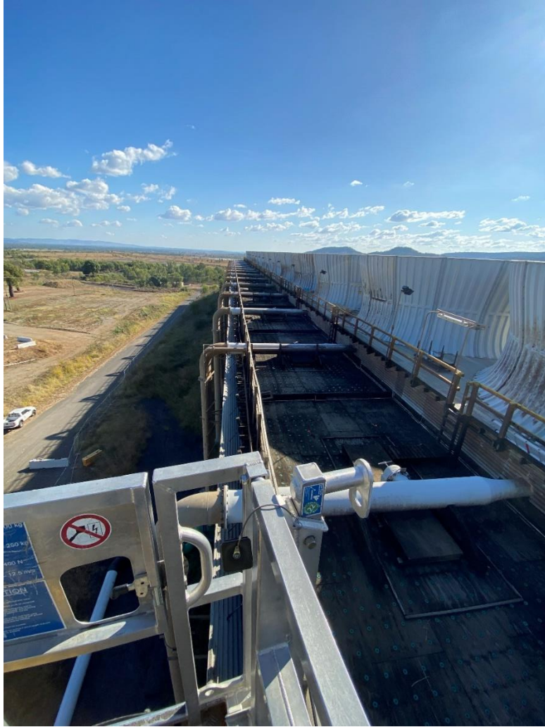
Figure 5.24 View of hot water basin. No evidence of sagging
