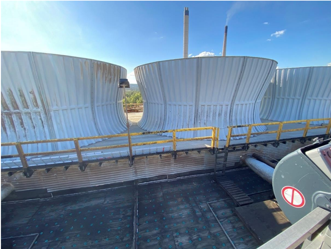
Figure 5.26 Fan deck appeared to be in good condition
